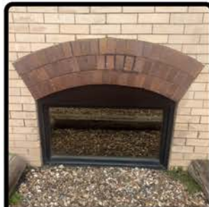
Brick Segment Arch
