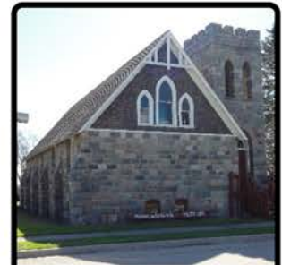
Cut Stone Walls
