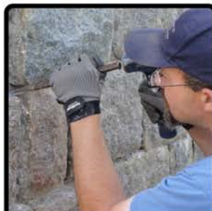
Masonry Repair (any)
